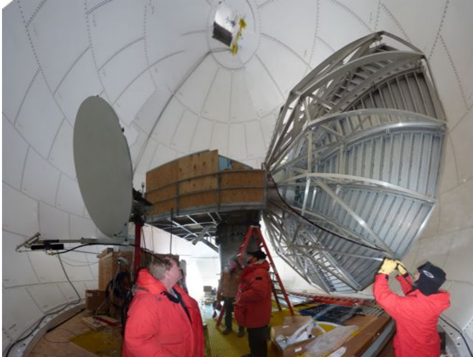
Figure 1: The 2.4m Skynet antenna (left) inside the 9m radome at the Pole RF facility, January 2012
